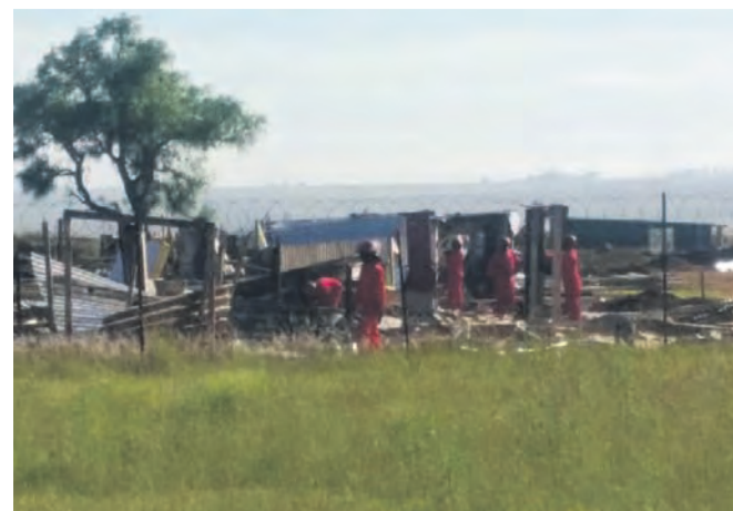
Red Ants Security Forces are breaking up alleged illegal structures at Skoonplaas Informal Settlement.
