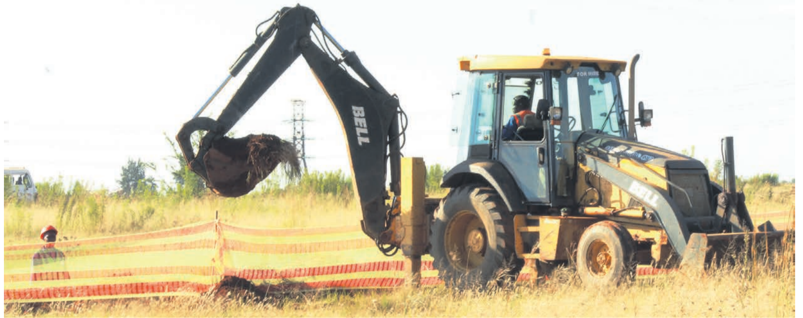
Construction at Payneville Extension Three started in January. Phase one includes the roads and storm water infrastructure, which will be completed in October.
